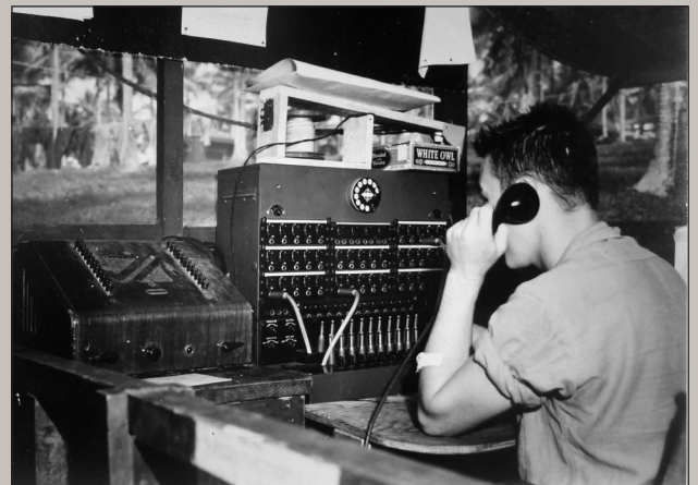
The telephone switchboard for Marine Corps Squadron VMD-154 in 1943. It handled communications traffic within the squadron's camp and out to the wider base area. Photo – US Archives.
