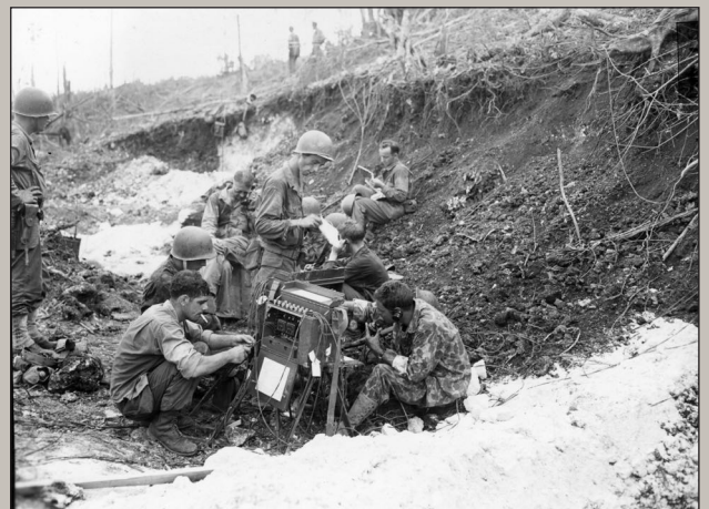
Speed was everything in combat. This telephone centre was set up two hours after landing at Kamiri Airstrip, Noemfoor Island, Dutch New Guinea. Photo – Signal Corps Archives Photostream - Flickr.
