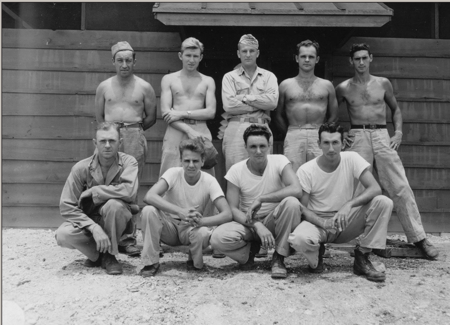
Installation Team 204 of the 71st ACS at Espiritu Santo. This job was to install critical early-warning radar systems, radio arrays, and fighter-control networks to guide Allied aircraft. Photo – Signal Corps Archives Photostream - Flickr.
