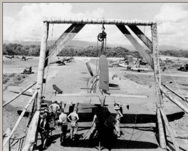
Boresighting the guns on a Corsair in a home-made frame constructed from coconut palms on Guadalcanal in 1943. Photo – US Archives.
