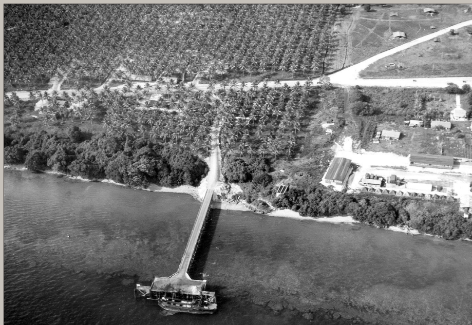
Base Button (Santo's) garbage pier as it was in 1943, complete with garbage ship ready to take on the base's refuse. The collection of buildings to the right is the Service Command Post Exchange. Photo – US Archives.
