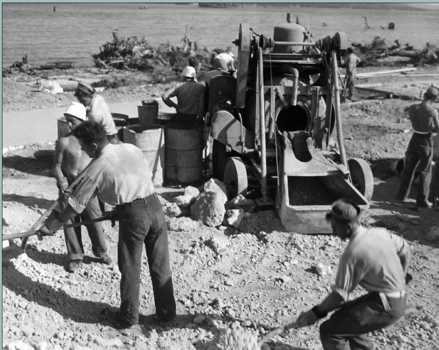
Men of 49th Seabees constructing 'runways' for torpedo trucks at what would become the torpedo repair shop on Santo. September 1943. Photo – US Archives.
