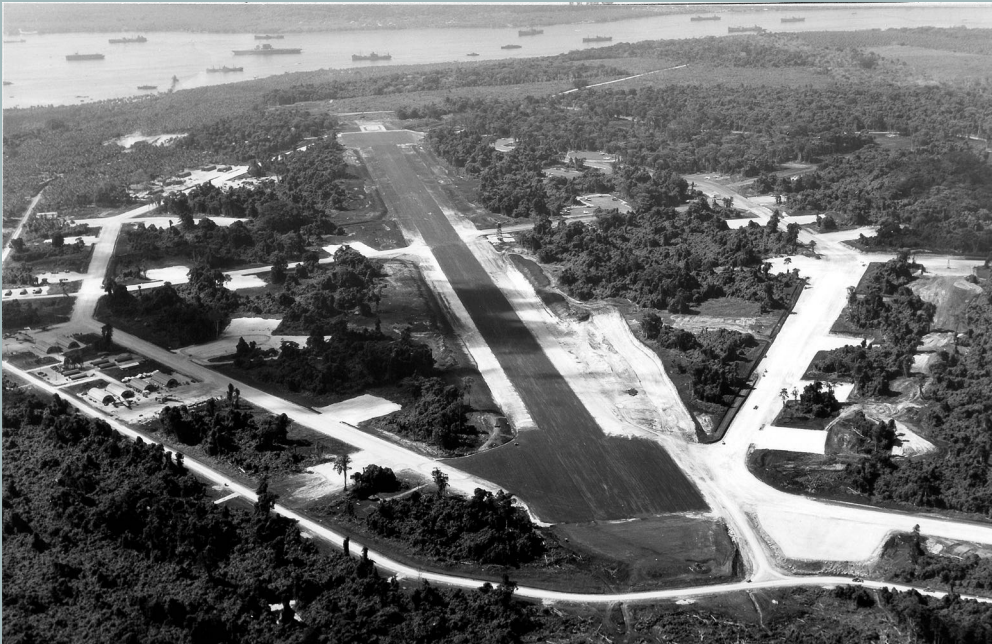
Bomber No.3 when it was the island's largest bomber base. Note the huge number of ships anchored in the Segond Channel at the top of the photo. The largest ship just to the left of the end of the runway is the aircraft carrier USS Saratoga. The narrow road heading on an angle towards the right from the end of the runway, is the road to the Catalina Seaplane Base on the Segond Channel. Photo – US Archives.
