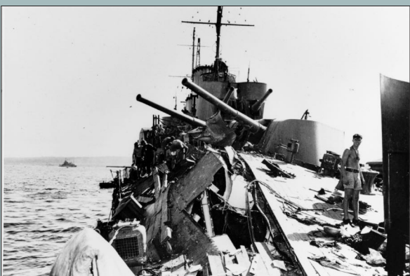
Hobart photographed on the quarterdeck, looking forward from about 207 frame port side, showing the ship's badly distorted aft deck and the after 6-inch gun turrets. Photo – U.S. Naval History and Heritage Command.
