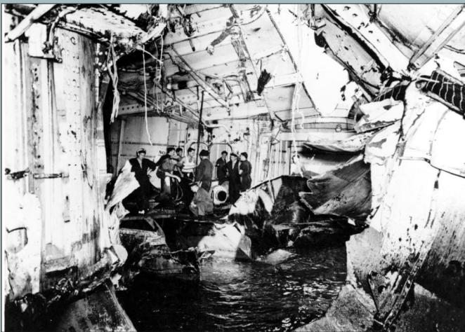
View taken at Espiritu Santo on 29 July 1943, showing damage inflicted when Hobart was torpedoed by a Japanese submarine on 20 July. Photographed looking aft from the centre line of the Ward Room from about 179 station, after clearing away the majority of the wreckage. Photo – U.S. Naval History and Heritage Command.
