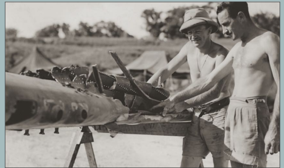
Two RNZAF ground crew standing by the wing of a P-40 Kittyhawk which is damaged on the leading edge. The muzzles of the .50 cal machine guns are at left. Guadalcanal, Solomon Islands. From Geoff Fiskin's personal collection. Photo – Masterton District Library.
