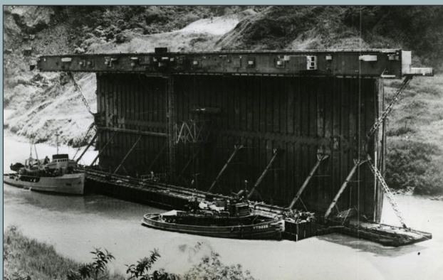
A US Navy floating dry dock section – turned on its side – makes its way through the Panama Canal's Culebra Cut, 18 July 1945. Photo – National WWII Museum.
