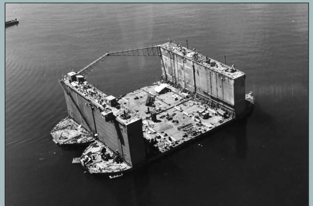
Wing walls are complete and in position on this pair of pontoons making up 20 percent of ABSD-1 in Pallikulo Bay. Photo – US Archives.
