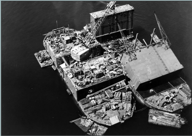
An aerial photograph of two of the pontoons in Pallikulo Bay being assembled. One wing wall has already been raised while a second is slowly being tilted into position. Photo – US Archives.
