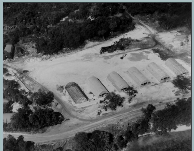
The Aviation Supply Depot's quonset huts under construction in 1943. Photo – US Archives.
