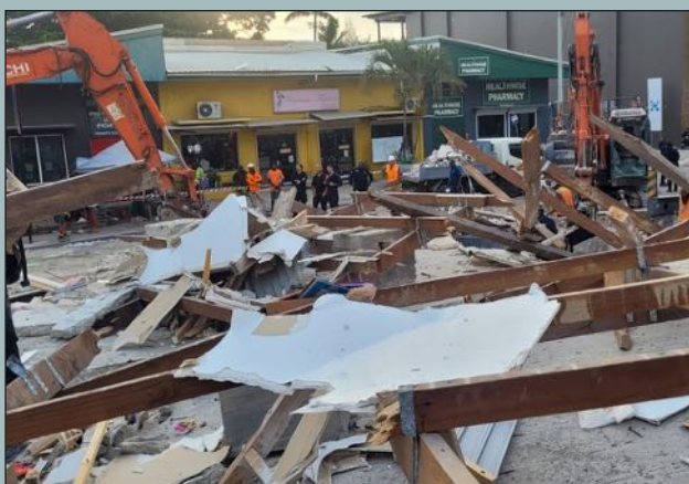
Damage to buildings and infrastructure in the capital Port Vila and surrounding areas was extensive. Power was out, water unavailable and all important communications were down. Photo – Various sources.
