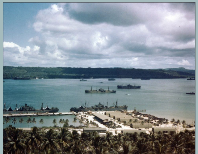
A rare colour photograph of the main wharf in what is now Luganville where the majority of Liberty ships were unloaded. Their cargo was then transported to some of the hundreds of Quonset huts and depots built all over the island.
