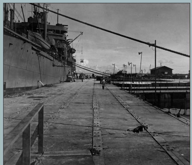
The floating pontoon wharf at Pallikuo Bay. This was where the Oriental was due to unload. Photo – US Archives.
