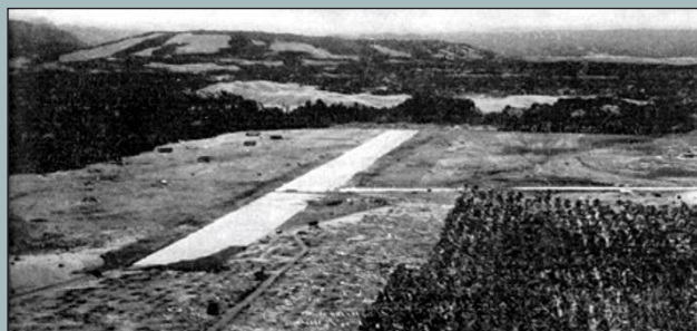
The airfield at Lunga Point on Guadalcanal, later called Henderson Field by the Allies, seen under construction by the Japanese in July 1942. Photo – Marines in World War II Historical Monograph, 1949.
