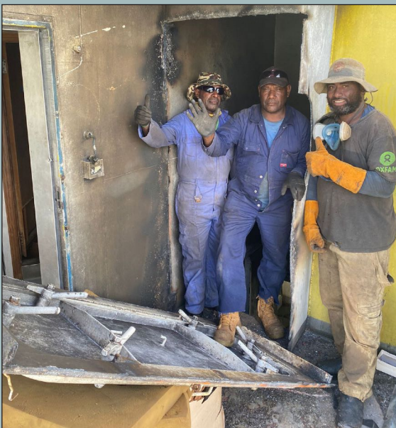
Thumbs up from the cutting crew for a job well done.
