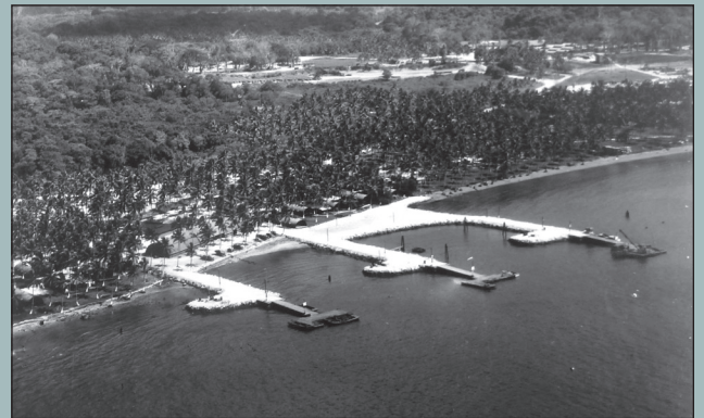
The three NATS piers built to the west of present-day Luganville on the Second Channel. Photo US Archives.
