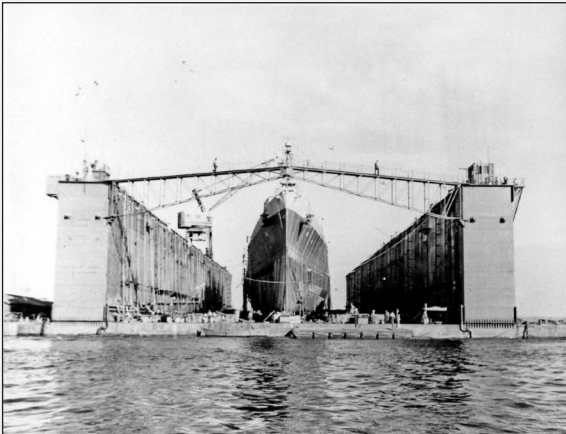
Not the Denver, but her sister ship the Columbia in the same floating dry dock in Espiritu Santo. Pic - US Archives.
