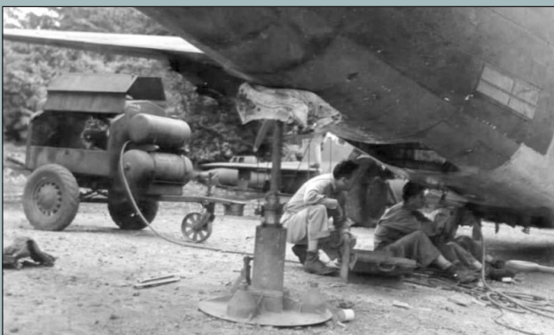
Repairing the skin of a Liberator bomber without a hangar full of the latest tools, spares and gear. Photo US Archives.
