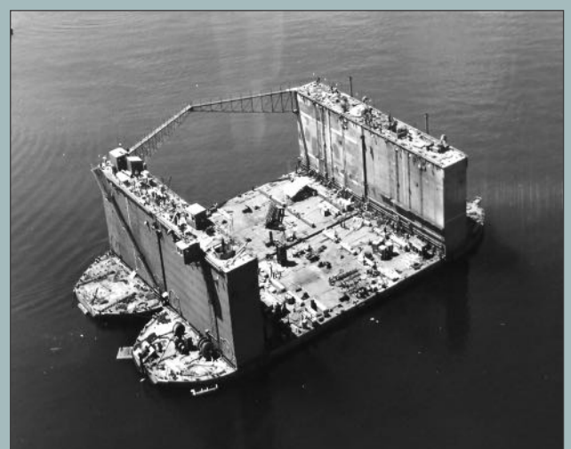
Two sections of ABSD-1 have had their 'wing walls' raised and welded into position in Pallikulo Bay. Photo US Archives.
