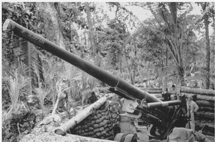
A 155mm Long Tom Gun M1. The gun could fire a 100 lb (45 kg) shell to a maximum range of 14 miles (23 km). A little less sophisticated than its more modern Ukrainian cousin, but just as effective.
