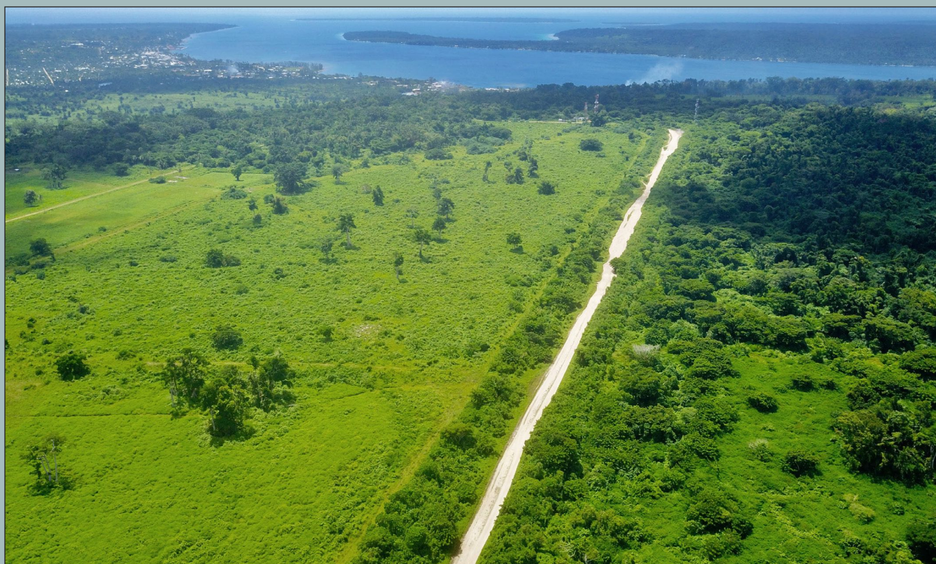
Bomber #3 Airfield as it is today. The runway has been turned into a road running across the plateau at the top of the hill. Towards the top left of the photo you can see Luganville in the distance. Photo Kevin Green.
