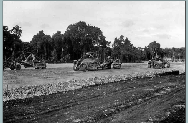
Caterpillar dozers pulling scrapers or 'carry-alls' level the thick coral base of the runway at Bomber #3. Photo US Archives.
