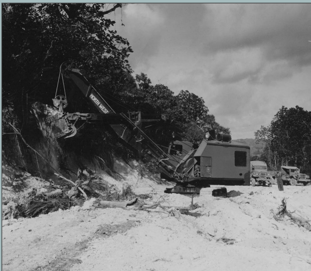
Massive quantities of coral had to be excavated to create the Bomber #3 runway and taxiways. Photo US Archives.
