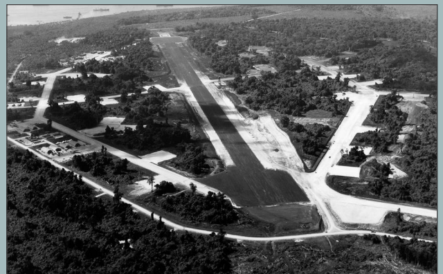
The completed Bomber #3 airfield with its asphalt coating which helped prevent gravel damaging aircraft. Photo US Archives. (continued...)
