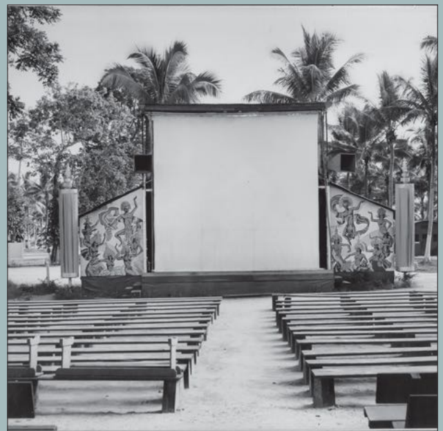
Some theatres on Santo were better than others. This very neat one was located at Hospital #6 on the island.
