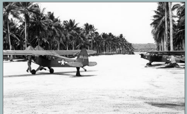
Sandberg Field in South Santo, bulldozed through a coconut plantation.
