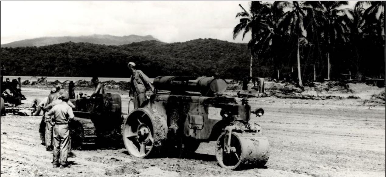
US Navy Seabees construct the runway at Segi Point, New Georgia.
