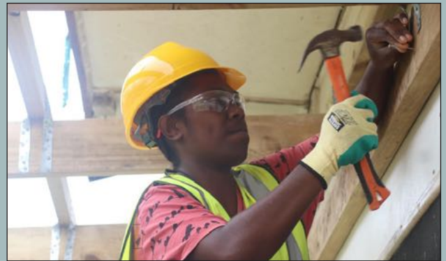
A carpentry student at work in Port Vila.
