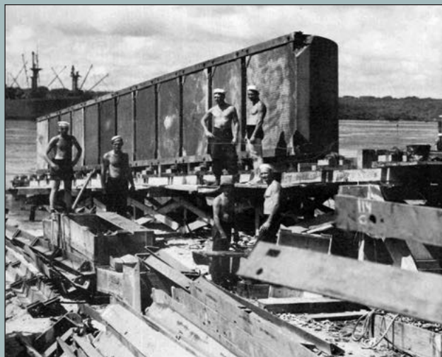
Seabees from the 40th Battalion stand next to many pontoons joined together to make up one big floating pontoon.
