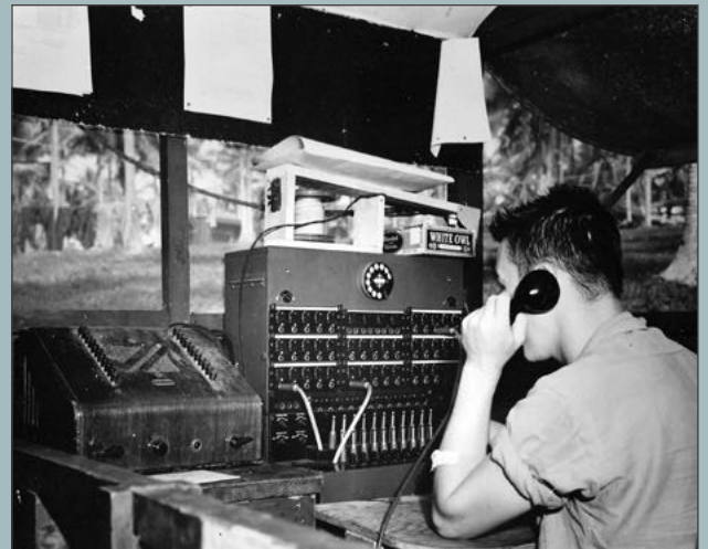
Telephone Switchboard at VMD-154 Camp Elrod, Espiritu Santo.
