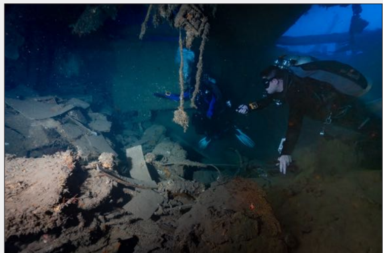
The collapsed swimming pool is inspected by divers from Pacific Dive. Photo Pacific Dive.
