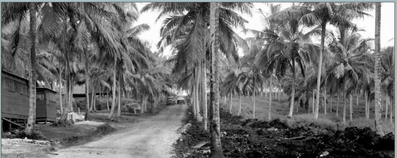
Road scene looking north from mess hall at VMD-154 Camp Elrod, Espiritu Santo.
