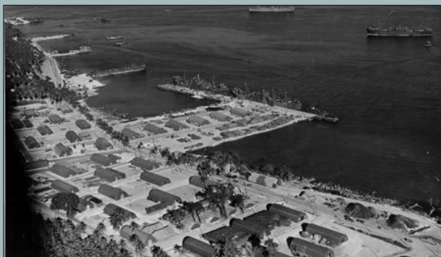
Part of the massive warehouse and supply depot on the foreshore at what is now Luganville. Picture - US Archives.
