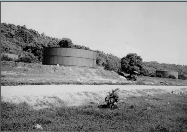
Some of the massive fuel storage tanks on Aore Island, just across the Second Channel from Espiritu Santo. Photo - US Archives.
