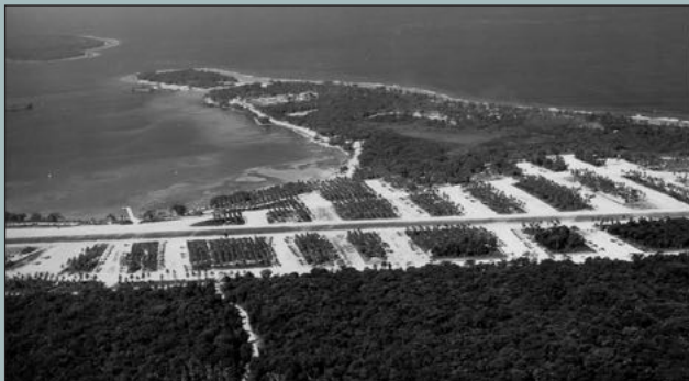
Bomber #1 or Pallikulo Airfield on Espiritu Santo was the first of the three bomber airfields built on the island. Photo - US Archives.
