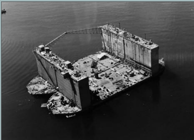
ABSD-1 undergoes assembly in Pallikulo Bay off Aessi Island. Photo - US Archives.
