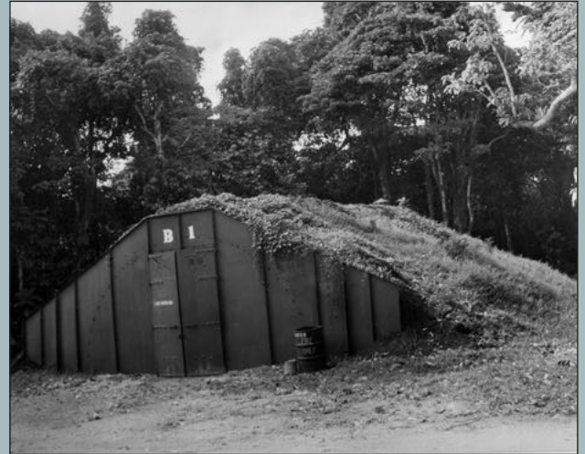
One of the many ammunition storage bunkers on Espiritu Santo. These are still visible today. Photo - US Archives.
