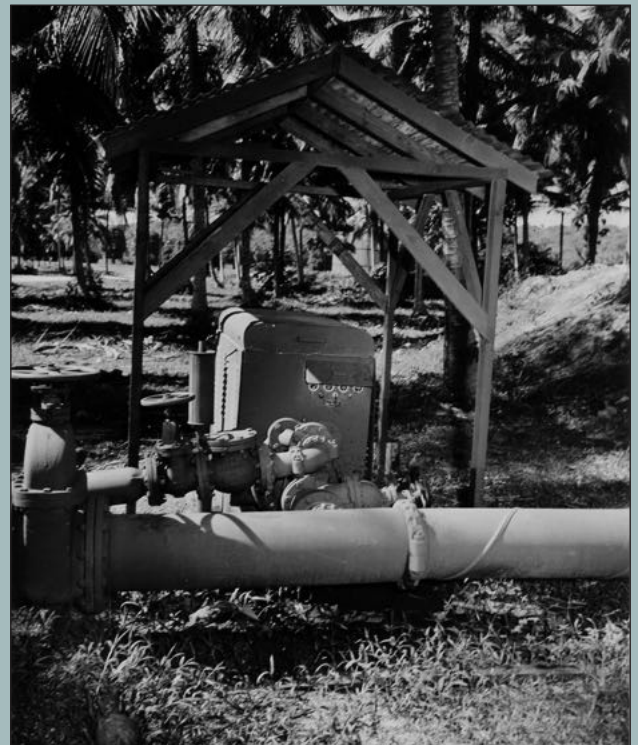
One of the large pumps used to transfer fuel to and from ships and the massive tank farm on Aore Island. Photo - US Archives.
