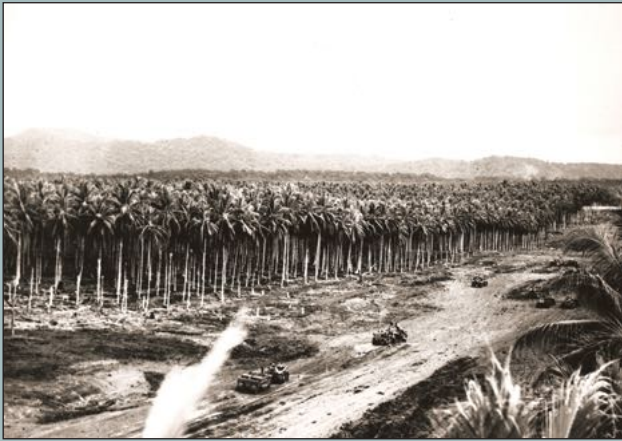
Construction of Henderson Field on Guadalcanal in the Solomon Islands was backbreaking work, carving the runways and taxways out of the coconut plantations and native jungle.
