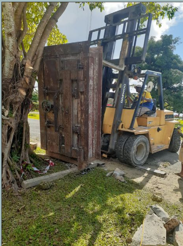
One of Santo Hardware's larger forklifts was used to unload the vault door and raise it into its vertical position oncemore.
