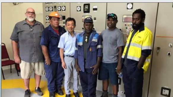
The Ambassador at Santo's hydroelectric power station.
