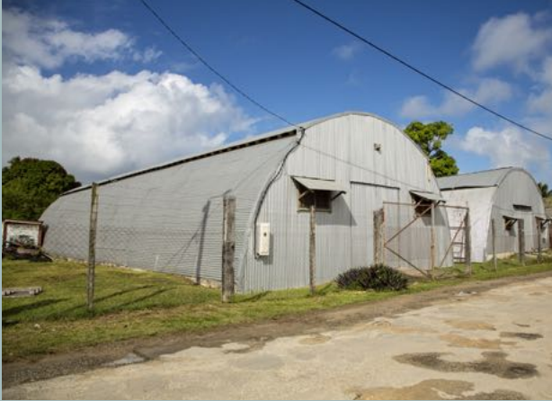
A pair of Quonset huts just off the main street in Luganville.
