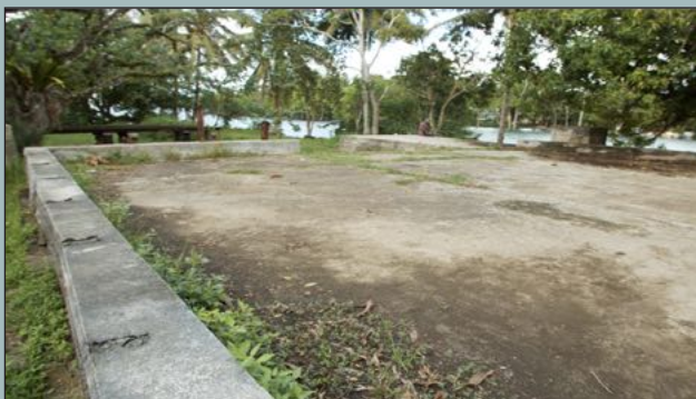
The slab upon which the Quonset hut would be rebuilt.
